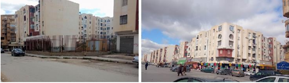
Fig. 3. 434 housing units (Source: Authors, 2022)
