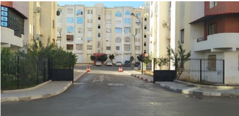
Fig. 11. The vehicular access gate has not yet been achieved (Source: Authors, 2022)
