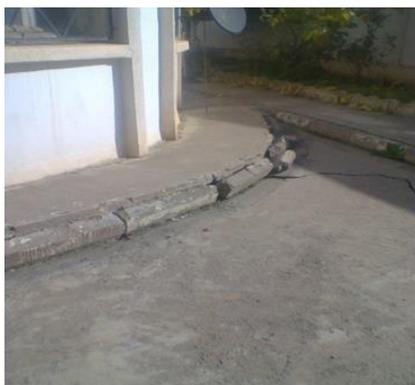
*Fig. 2. Effects of landslides on the sidewalk (source: Prepared by Authors with cam program, 2022)*
