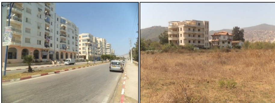
Fig. 10. Residential development at the expense of farmland on Bejaia periphery
