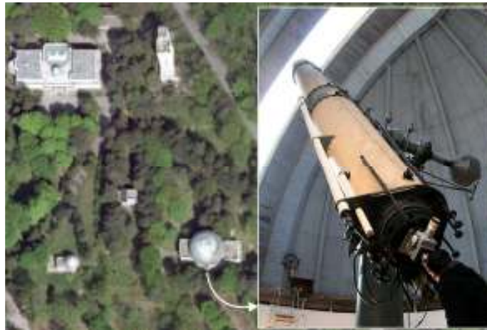
Figure 1. Ortophoto capital given the complex Astronomical Observatory (Administrative building, top-left) and photos of the Great refractor (right)
