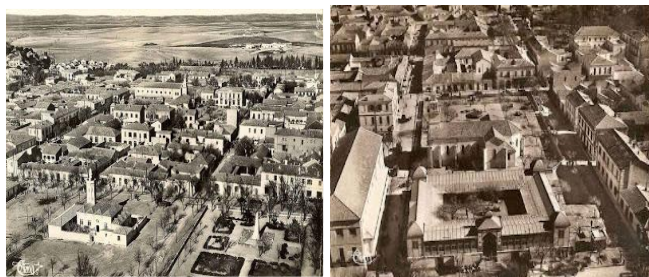
Fig. 3. The orthogonal layout of the roads in the colonial center of the city of Ain-Beida (Source: Ain beida history. Blogspot.com/p/blog-page_6.html)
