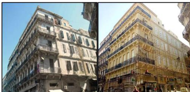
Fig. 10. Rehabilitated building located on Med Khmisti Boulevard (Source: OPGI Oran)
