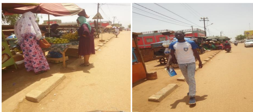
Fig. 4. Pedestrian crossings occupied by fruit and vegetable vendors (Soma et al., field observation, June 2022)
