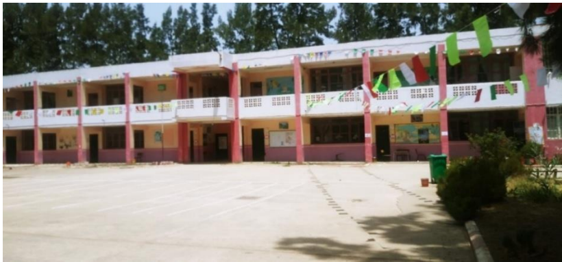
Fig. 5. A general view of classrooms block. Source: Authors
