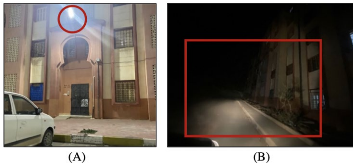
Fig. 8. (A) Lighting of block entrances, (B) Total absence of exterior lighting
