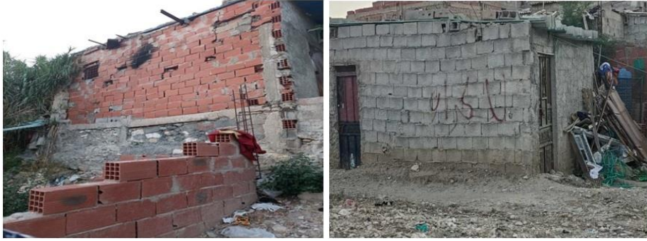
Fig. 7. Distribution of roofing materials in precarious housing (Corrugated metal and fiber cement) in El Zaouia (Field Survey, 2023)
