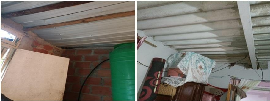
Fig. 8. Use of construction materials for housing envelopes (Brick and Cinder Block) in El Zaouia (Field Survey, 2023)
